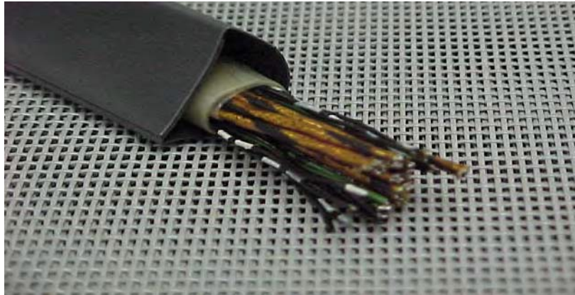
Photo 4: PRT aligned over Z-block Tape
