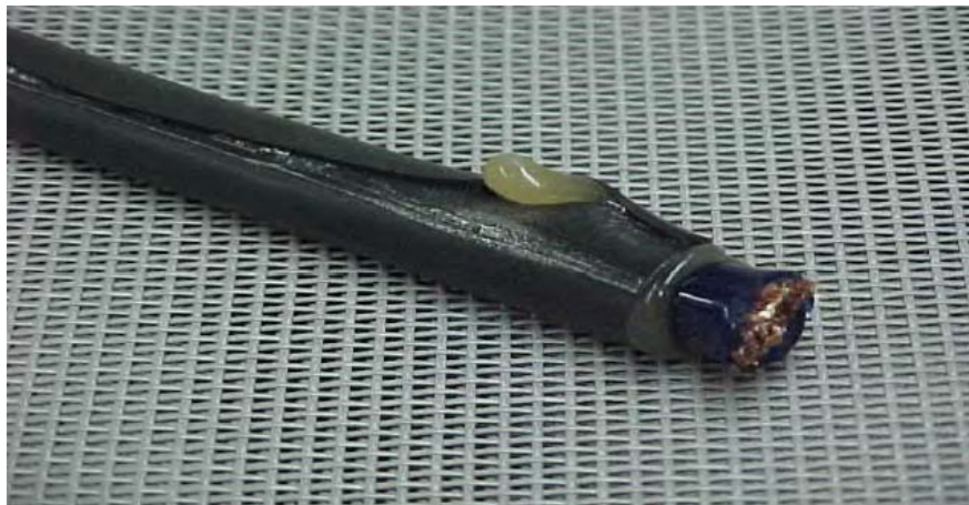
Photo 15: Seam rupture; too much heat, too fast!
