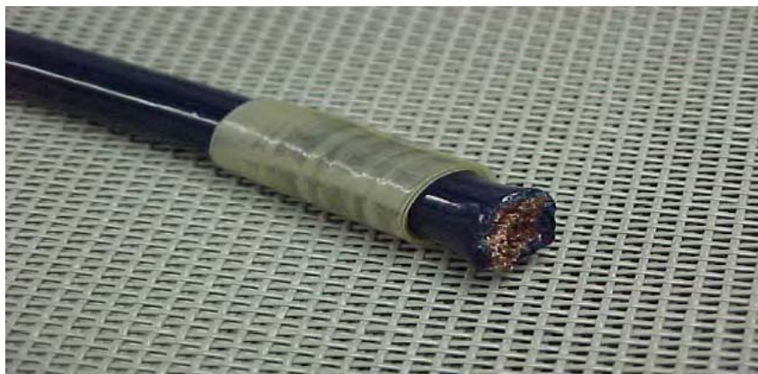
Photo 8: Z-Block tape wrapped around cable
